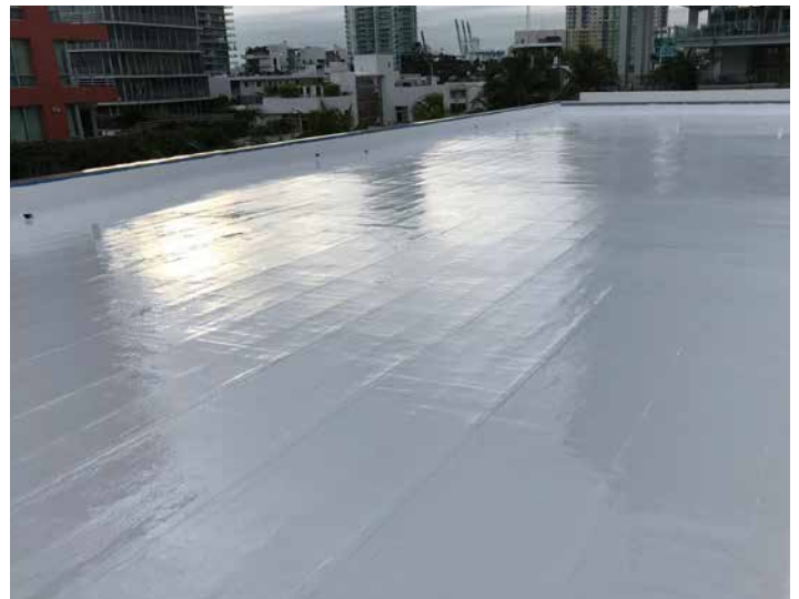
7870 HSS topcoat on a modified bitumen roof
