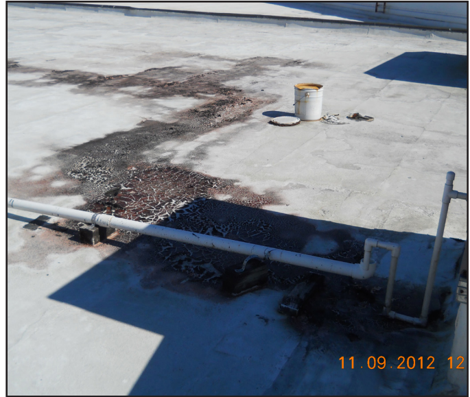
Poorly maintained condensate drain lines
