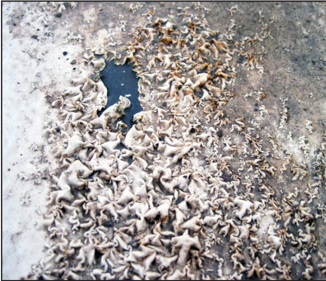
Delamination due to thin topcoat and ponding
