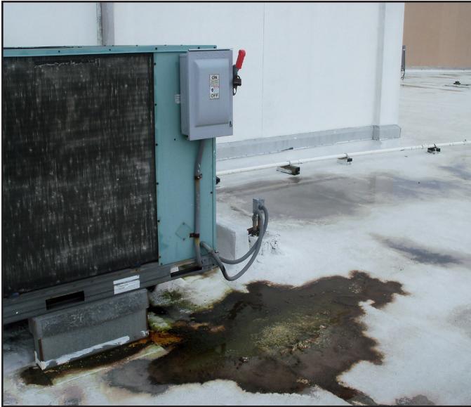
Disconnected condensate drain lines
