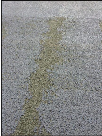
Delamination due to incompatible materials
