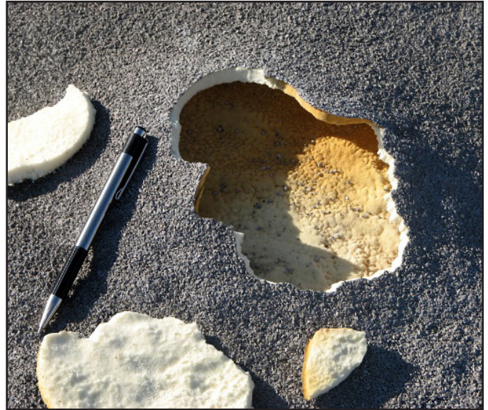
Foam blister that has been cut open
