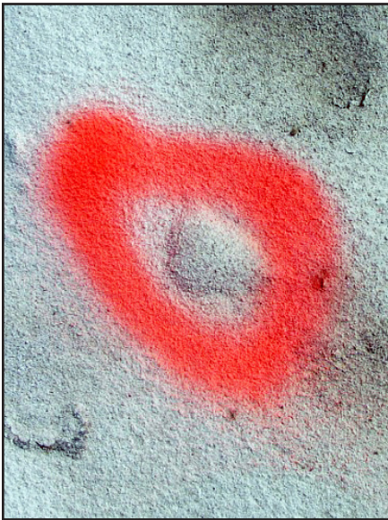
Blister due to contamination
