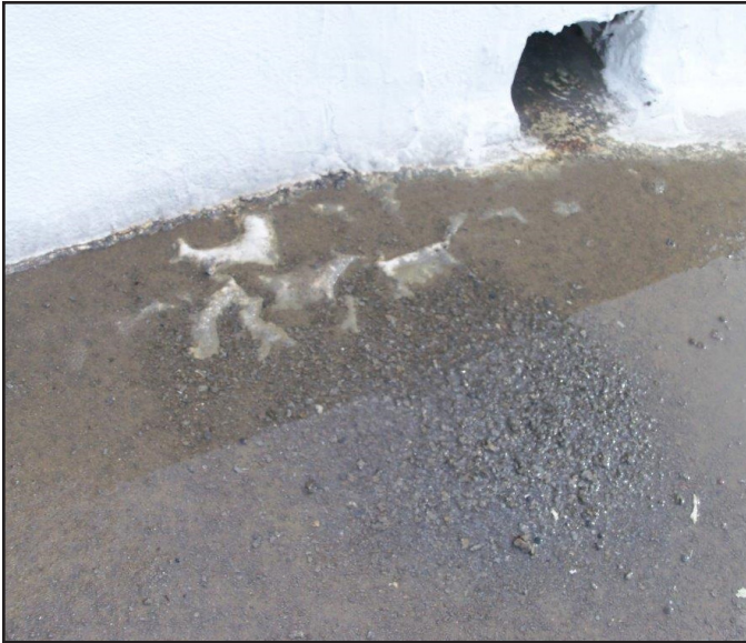
Scupper installed too high
