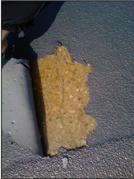
Delamination due to moisture
