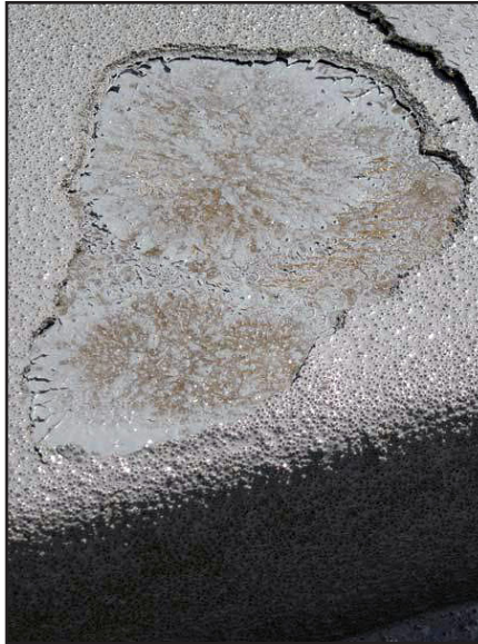
Area underneath removed blister
