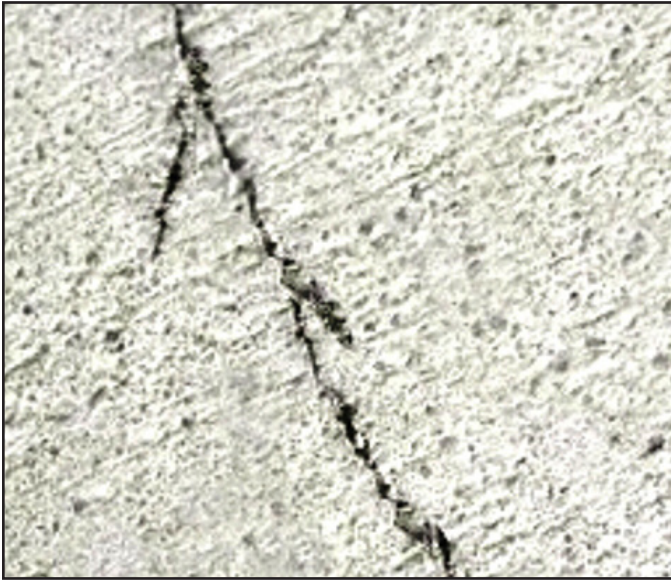
Crack before coating
