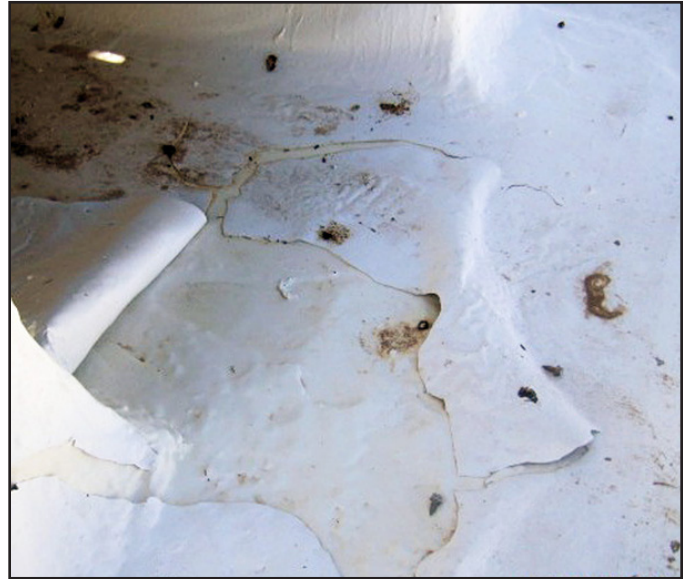
Delamination due to improper cleaning
