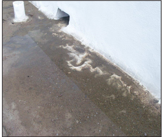
Clogged roof drain
